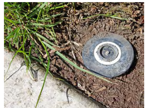
Figure 15. Pop-up rotors deliver water to the home lawn without interfering with foot traffic and equipment.
