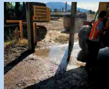
Vehicle wash water should not flow off washpad or discharge to the ground
