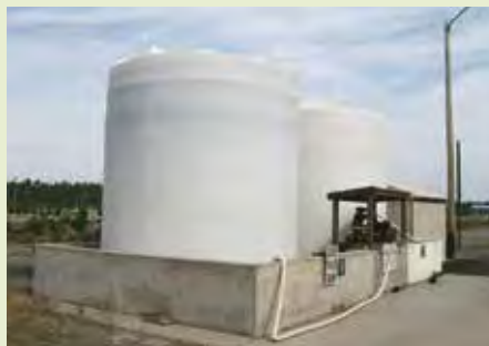
Concrete containment
