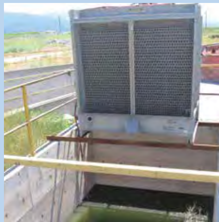
Approved wastewater retention pit with mechanical evaporator
